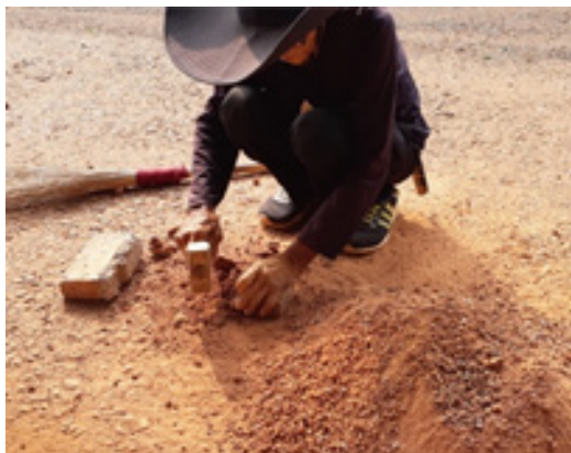
Figure 6. Rubble refinement process (source: processed by researchers)
