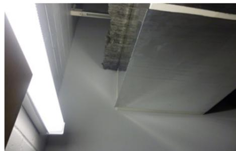
Figure 11. Air Conditioning Ducting Penetrate The Partition from The Receiver Room to The Source Room
