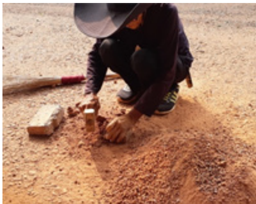
Figure 6. Rubble refinement process (source: processed by researchers)
