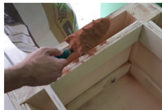
Figure 7. The process of adding fine aggregate (source: processed by researchers)
